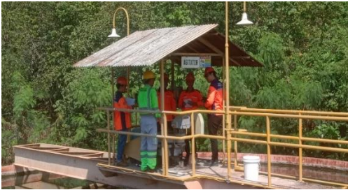
Gambar 3. Repairing teknologi watertreatment
